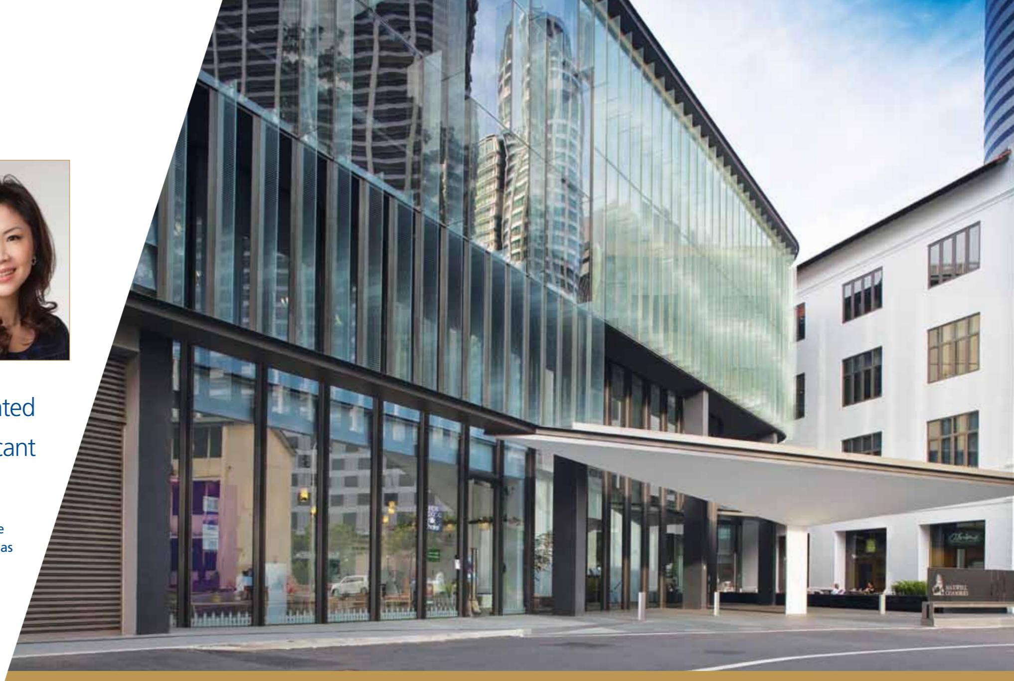
Entrance to Maxwell Chambers
